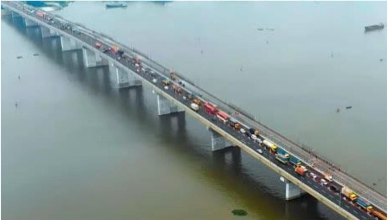
2nd Meghna Bridge on May 2019
